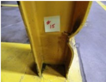
If the flange is damaged, the column can be repaired with flange replacement.
